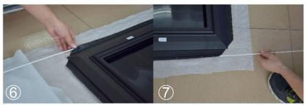
Insert the support bars into the four sides of the fabric.
